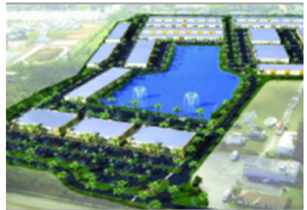
The 595 Park of Commerce in Davie has a 50,200-square-foot building under construction.
